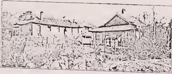
Kunsan Hospital Buildings.
